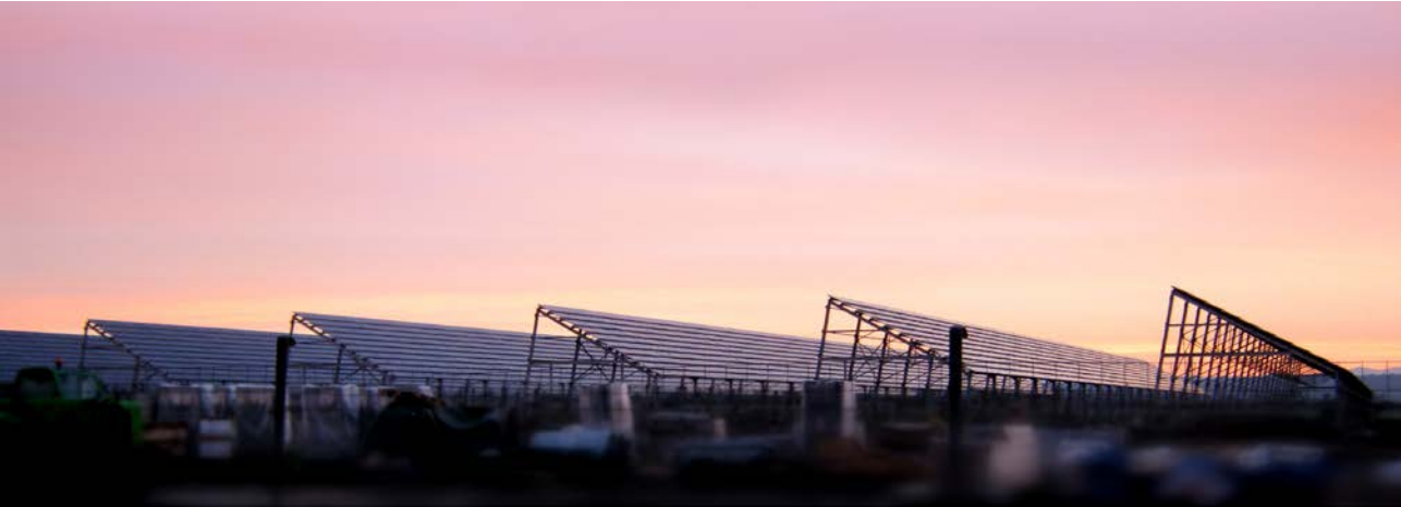
12 MW PV Plant Sardinia Italy 🇮🇹
