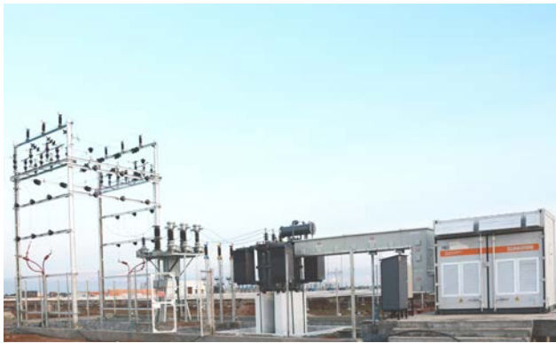
50 MW PV Plant India 🇮🇳
