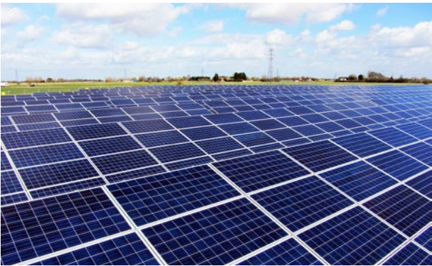
13.03 MW PV Plant UK 🇬🇧
