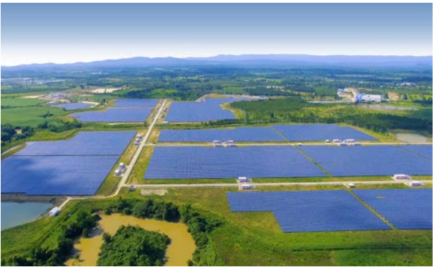
40 MW PV Plant Thailand 🇹🇭
