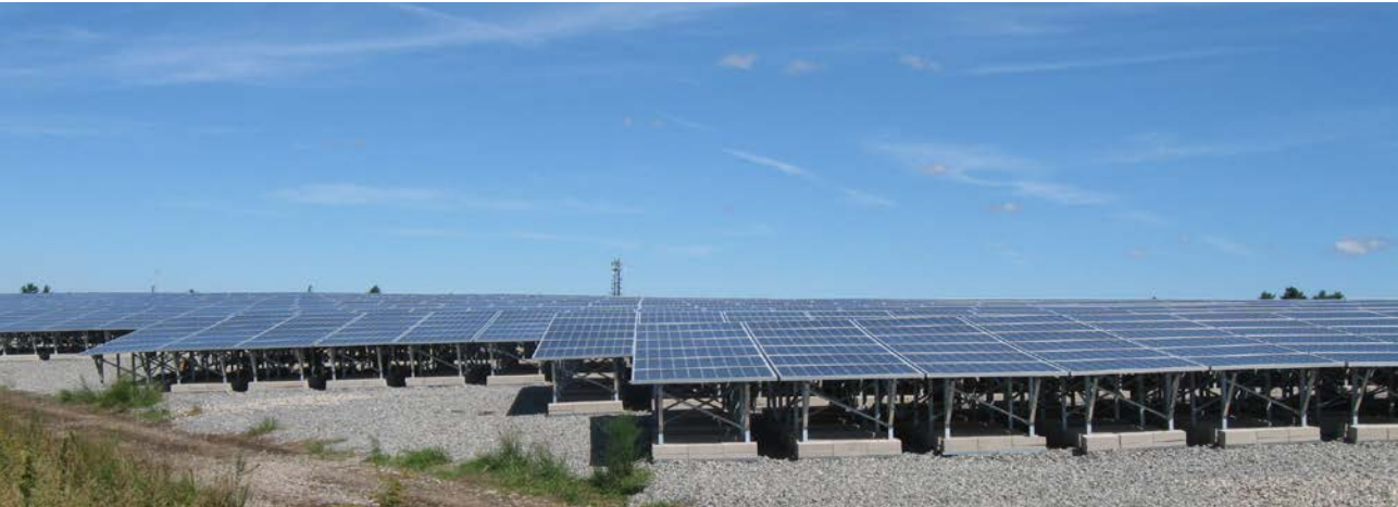
5 MW PV Plant Carver USA 🇺🇸
