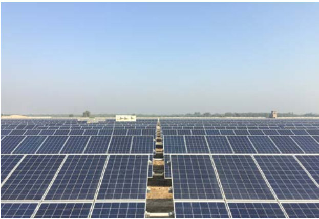
225 MW PV Plant Pakistan 🇵🇰
