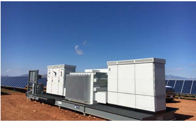
30 MW PV Plant USA 🇺🇸
