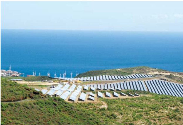
5 MW PV Plant Spain 🇪🇸
